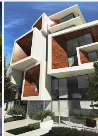
APERTURE - SOUTHWEST CORNER
